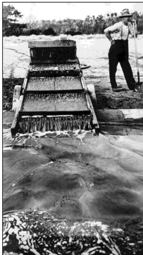
Figure 5-9. Man operating gold-saving tables at Nine Mile beach (Unknown, 1900).
