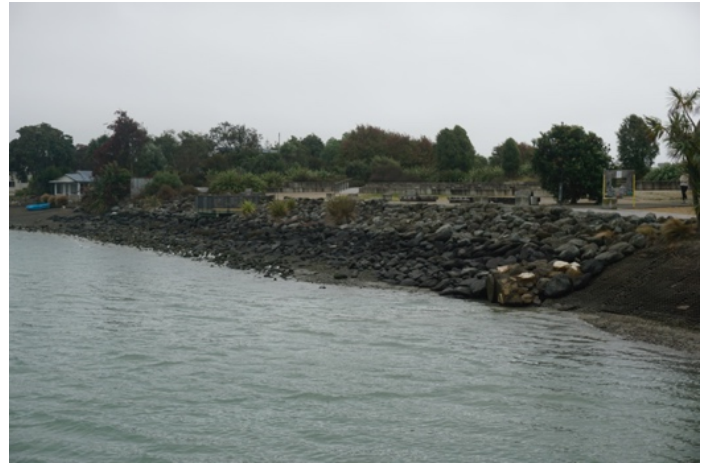
Figure 65: Images showing smaller engineered sea walls along the coastline of Māpua (Hubert, 2022b)
