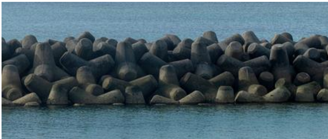
Figure 6.12: Tetrapod blocks forming a breakwater offshore of Ogimi Village on the north eastern side of Okinawa Island, Japan (Masucci et al. , 2019).
