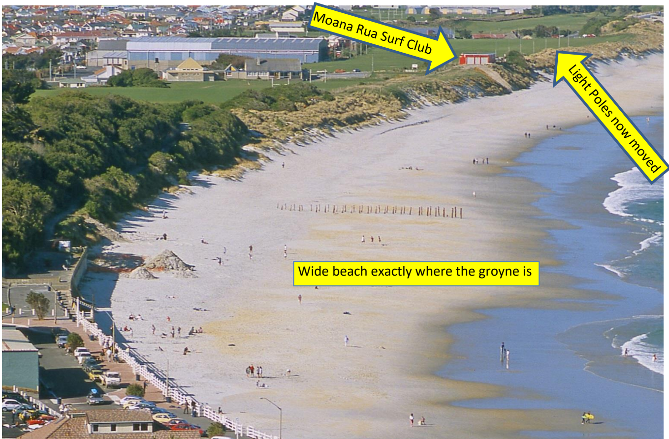
St Clair 7 , late 1980's showing Moana Rua Surfclub (demolished 2001). The dunes are now further back than the light poles which were undermined by waves. New poles were installed 10m further inland and are now under threat. The land under the surfclub has been completely lost to the sea. Note sand accumulation exactly at the groyne.
