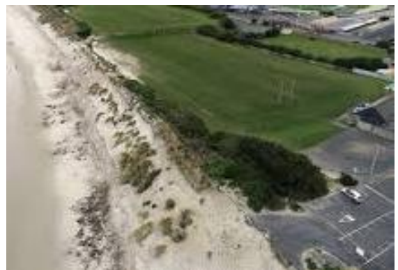
Below is a similar angle from 2019 showing another 10 metres of sandhill and asphalt lost.
