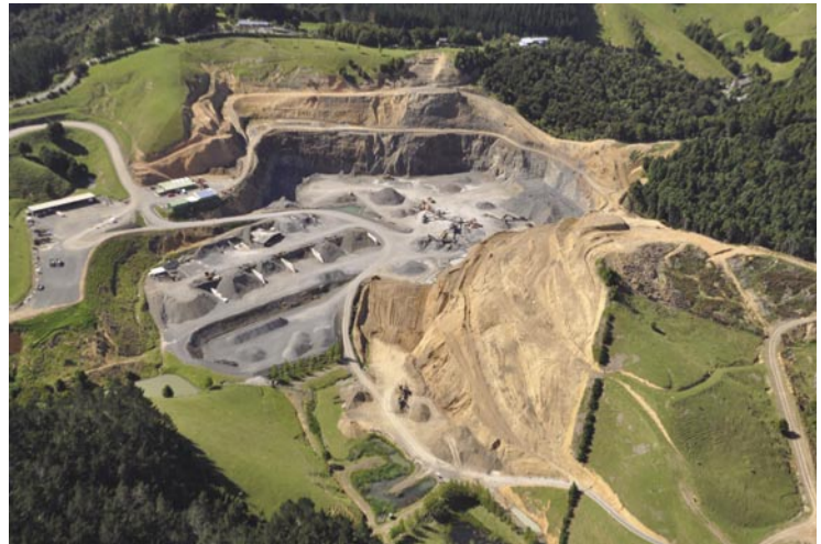
12.1 The 5-20 m-thick orange clay that overlies fresh blue-grey greywacke in the Glenbervie Quarry, Whangarei, indicates the extent of deep weathering that has occurred in northern New Zealand.
