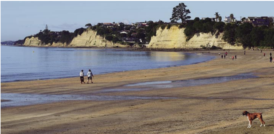
11.74 Eroding sandstone cliffs: The east coast of Auckland from Beachlands to Warkworth consists of rapidly eroding, near vertical cliffs of Waitemata Sandstone separating a series of small sandy beaches, each of which fills the mouth of a small drowned stream valley. The width of the shore platforms in front of the cliffs indicate cliff retreat rates of 1-3 m/100 yr. View south from Browns Bay, North Shore.
