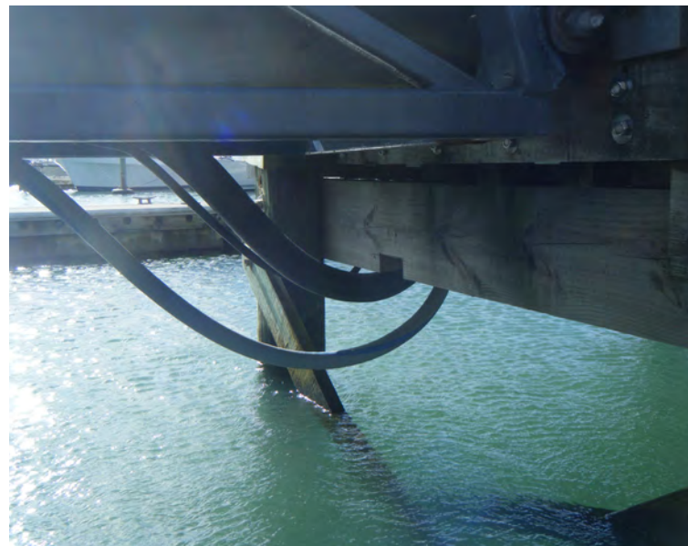
Figure 4.15 (bottom right): Junction of materials between the fixed timber wharf and moving metal bridge. Photographed by Sam Baxter, 2012.
