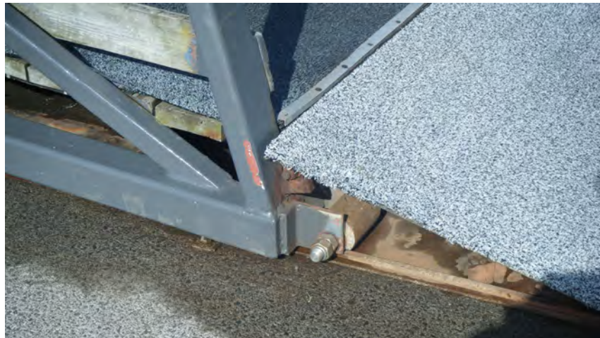
Figure 4.21 (bottom left): sliding ramp at Halfmoon bay that moves horizontally as the tides fluctuates. Photographed by Sam Baxter, 2012.
