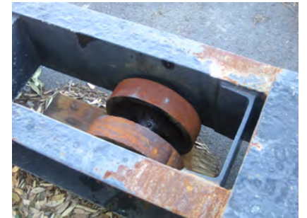
Figure 4.21 (bottom left): sliding ramp at Halfmoon bay that moves horizontally as the tides fluctuates. Photographed by Sam Baxter, 2012.
