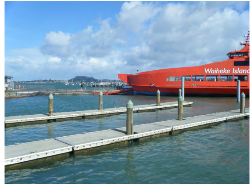
Figure 2.28 (above): Halfmoon Bay. The three rows of jetties form the lanes for the six boat ramps at Halfmoon Bay. In the Background the Sealink car ferry is docked on the concrete ramp at Susbrisky's Point. Photographed by Sam Baxter, 2012.
