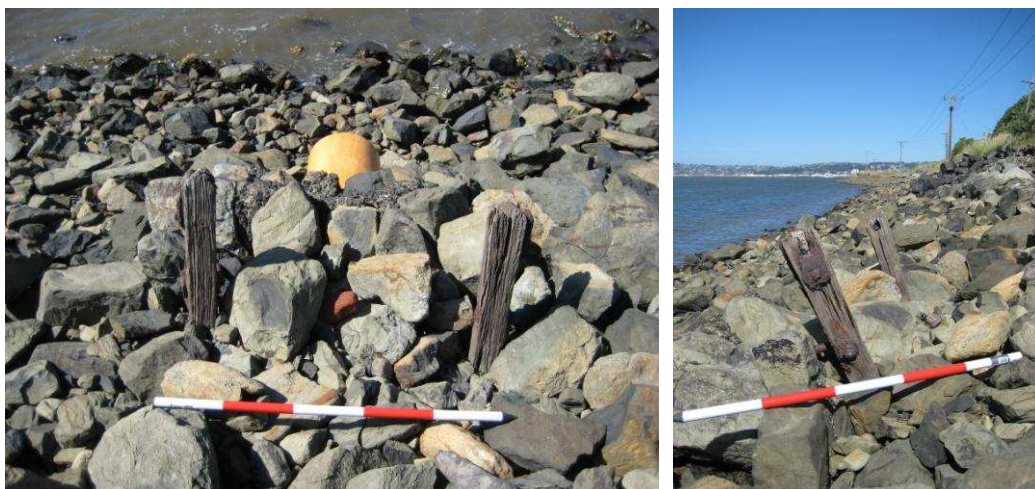
Figure 14: Photograph of Site 1 showing wooden culvert framing.
