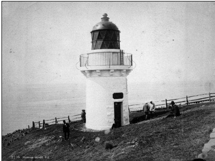
Figure 53: Taiaroa Head Lighthouse ca. 1890 (Alexander Turnbull Library (ref. PA1-o-287-47)).
