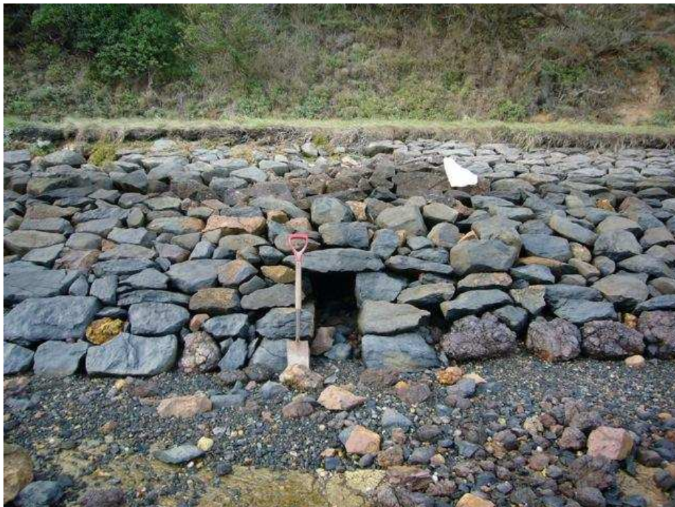
Figure 106: 1920s seawall built of slabby basalt later repaired in the 1950-70 period (photograph courtesy of Jill Hamel).
