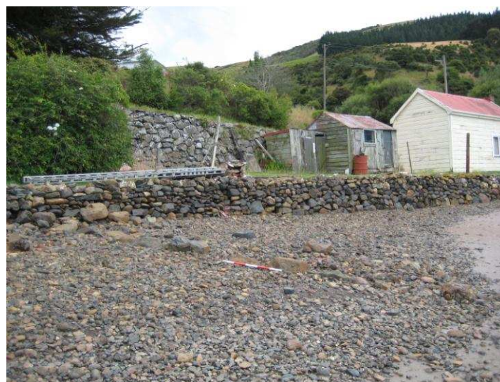
Figure 42: Photograph of Site 25 showing remains of small wooden pier.
