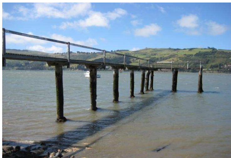
Figure 16: Photograph of Site 3 showing wooden jetty.
