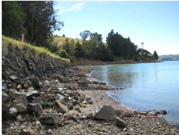
Figure 41: Photograph of Site 25 showing artificial boat landing area.
