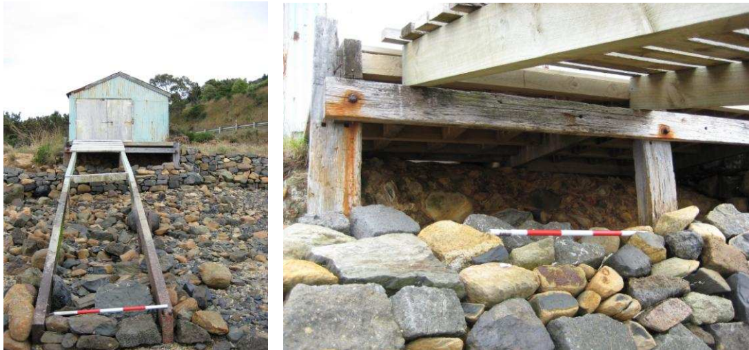
Figure 19: Photograph of Site 5 showing boatshed and slipway.
