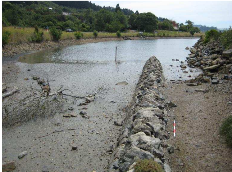
Figure 21: Photograph of Site 7 showing stone groyne.
