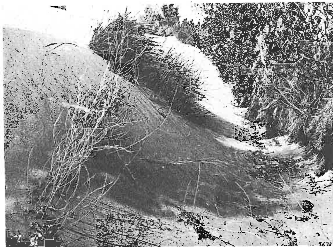
NO. 29. CATCHING-FENCE IN PROCESS OF BEING BURIED. DUNES, CROMWELL. FENCE ORIGINALLY 15 FT. TALL.
