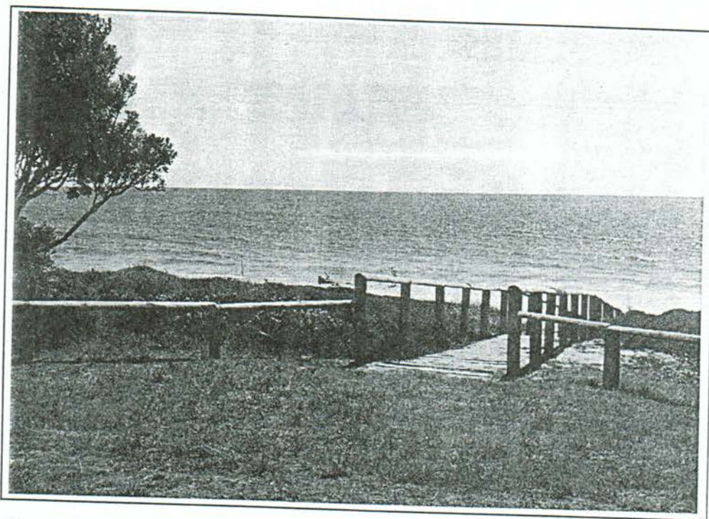
Figure 2b Completed walkway and associated post and rail fencing.
