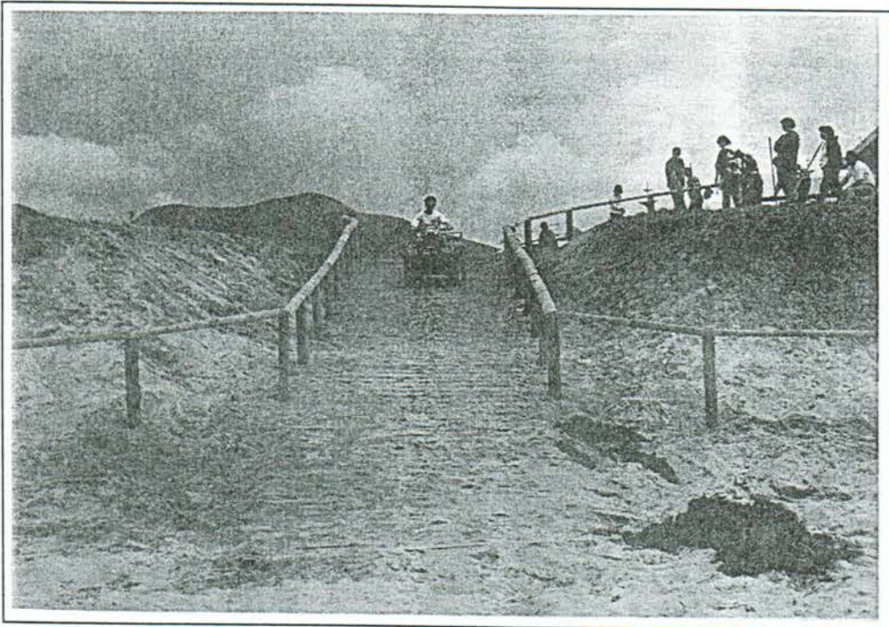
Figure 3b 'Testing' the newly constructed vehicle access-way.
