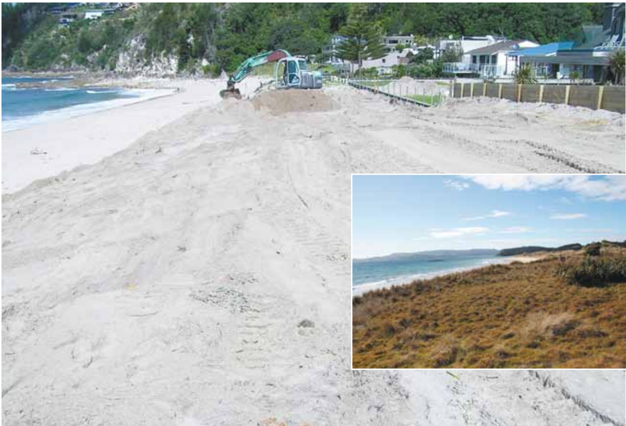
The 'whole of dune' approach involves mechanically removing the dense weedy layer from the dune (inset) to leave clean loose sand to allow planting of native sand binders on the foredune zone and native backdune species on the landward zone.
