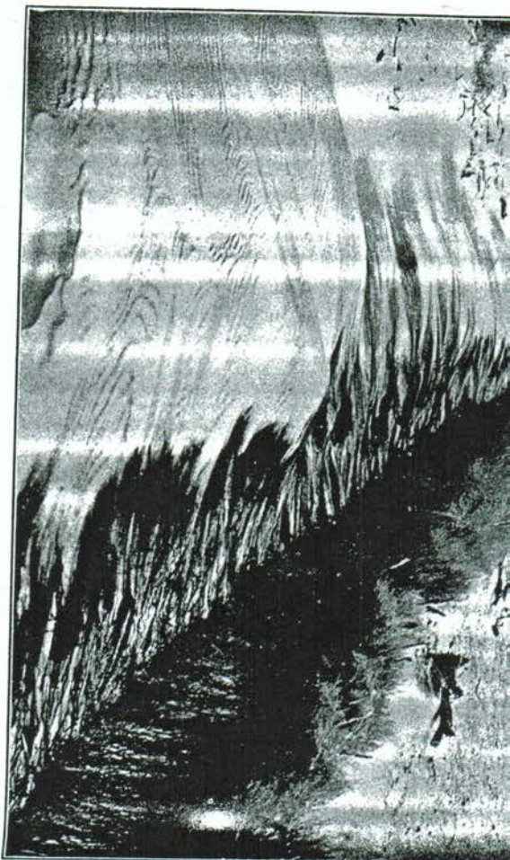
PLATE 1 Light permeable screen made of Manuka branches and No. 8 wire, showing the accumulation of sand to the lee of the screen. Waitare Sand Dune Reclamation Scheme. (Courtesy Soil Conservation and Rivers Control Council, N.Z.)
