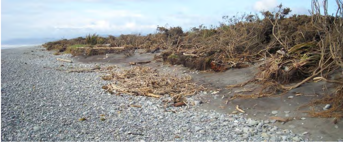
Figure 4.8. Landward erosions north of the New River Bridge (27/11/2011)
