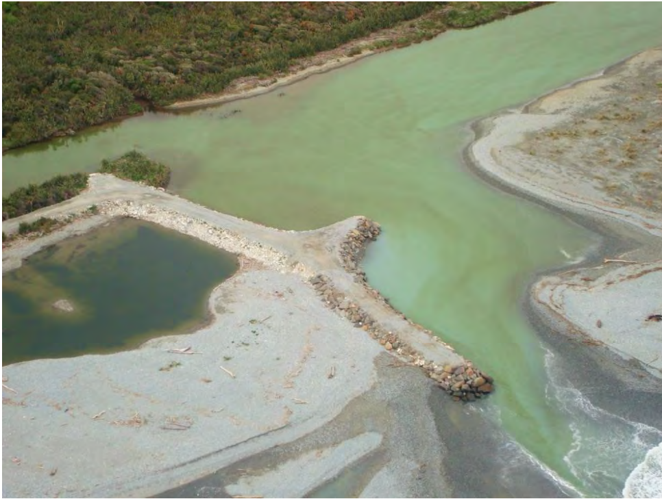
Figure 1.6. Artificial lagoon outlet and rubble-mound breakwater at the confluence of New River and Saltwater Creek (photo courtesy of Laurie Anderson, 23/05/2011)
