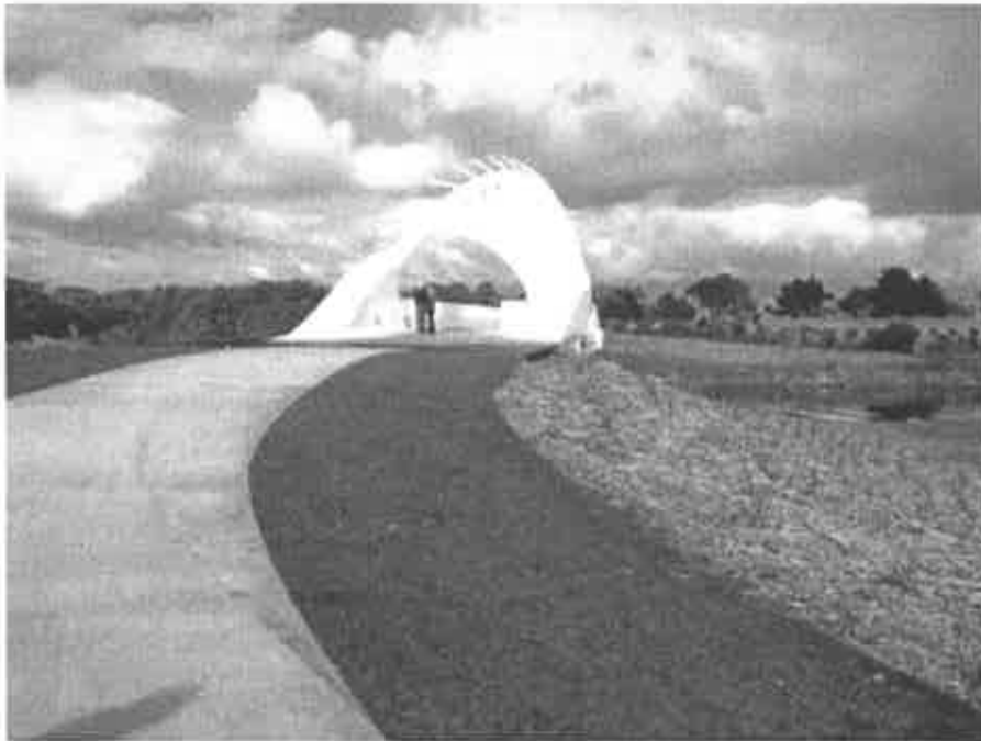
Figure 1. Te Rewa Rewa bridge just east of planting site.
