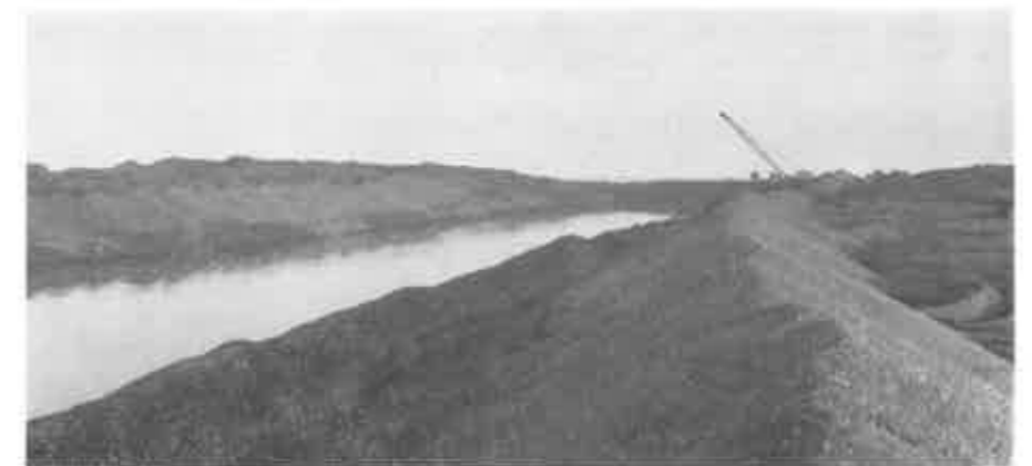
Figure 3 Cutting the channel through the spit at dusk, 28 June 1972. Photo W. G. Nealy, Ministry of Works
