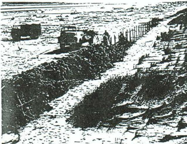
Simple foredune fence constructed of posts and thinning/pruning slash.
