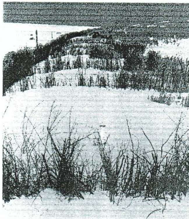
Photo 1. Willow-twig wind screens at the foot of the dune slope.
