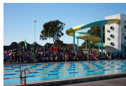
Powerco Aquatic Centre Outdoor Pool and Hydroslide
