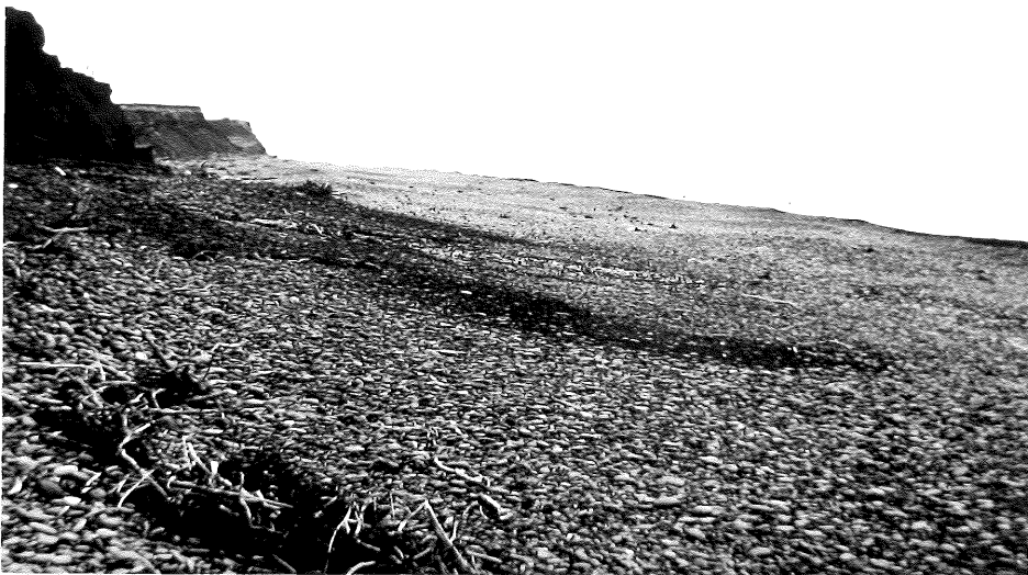
Plate 15. Clearance of the cliff debris at longbeach. 23/2/67. Erosion of the profile has removed all cliff debris as far landward as the storm berm.
