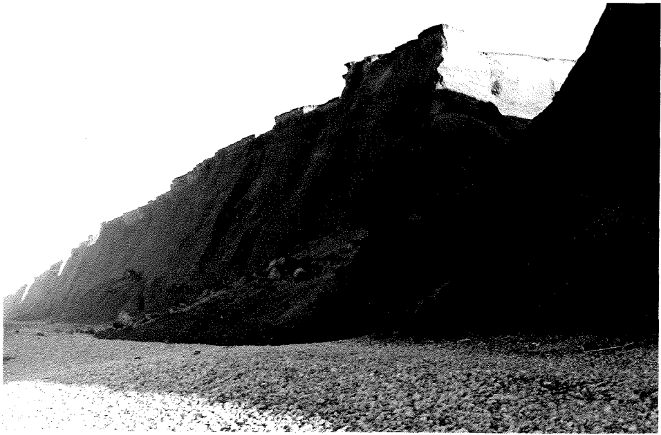
Plate 3. Prominent cliff-falls at Profile 12. Failure of the cliff-face occurs along clearly defined shear planes and leads to parallel retreat of the face and the maintenance of steep slopes.
