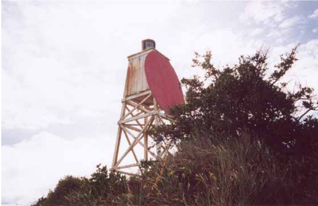
Navigation marker/light at Karaka Street, Wanganui (Castlecliff) from seaward. Photo: Tony Woodbury
