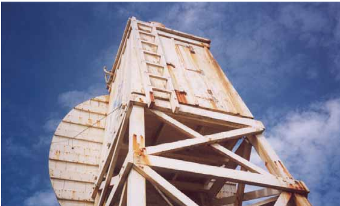
Close-up of the structure of the marker beacon at Karaka Street, Castlecliff, Wanganui (rear view). Photo: Tony Woodbury
