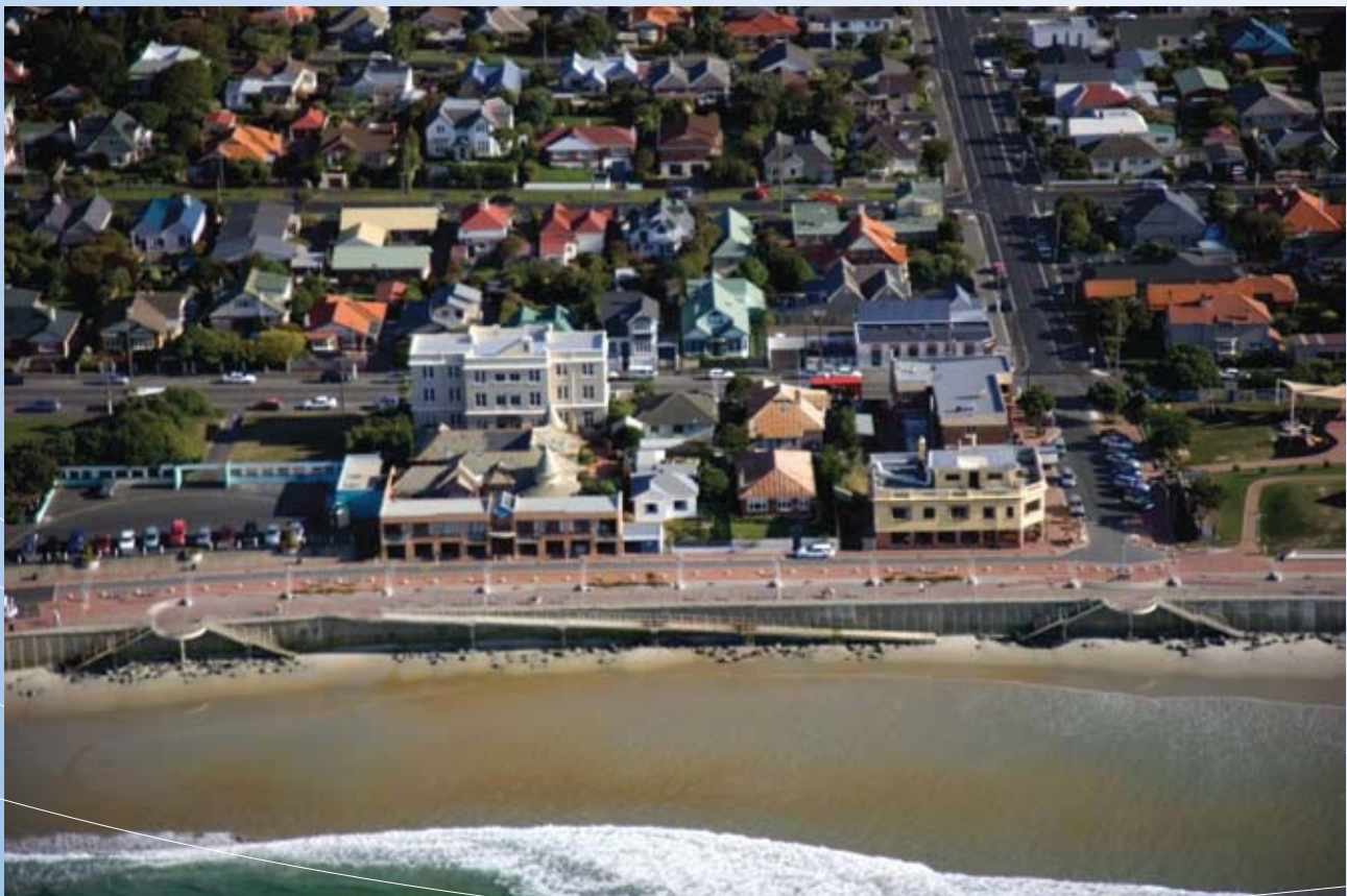
Figure 10. Concrete protection wall at St Clair. Structures like this along the coast will need to be strengthened to combat ongoing rise of sea level and higher storm surges, but will be expensive if valuable inland housing and infrastructure is to be protected.
