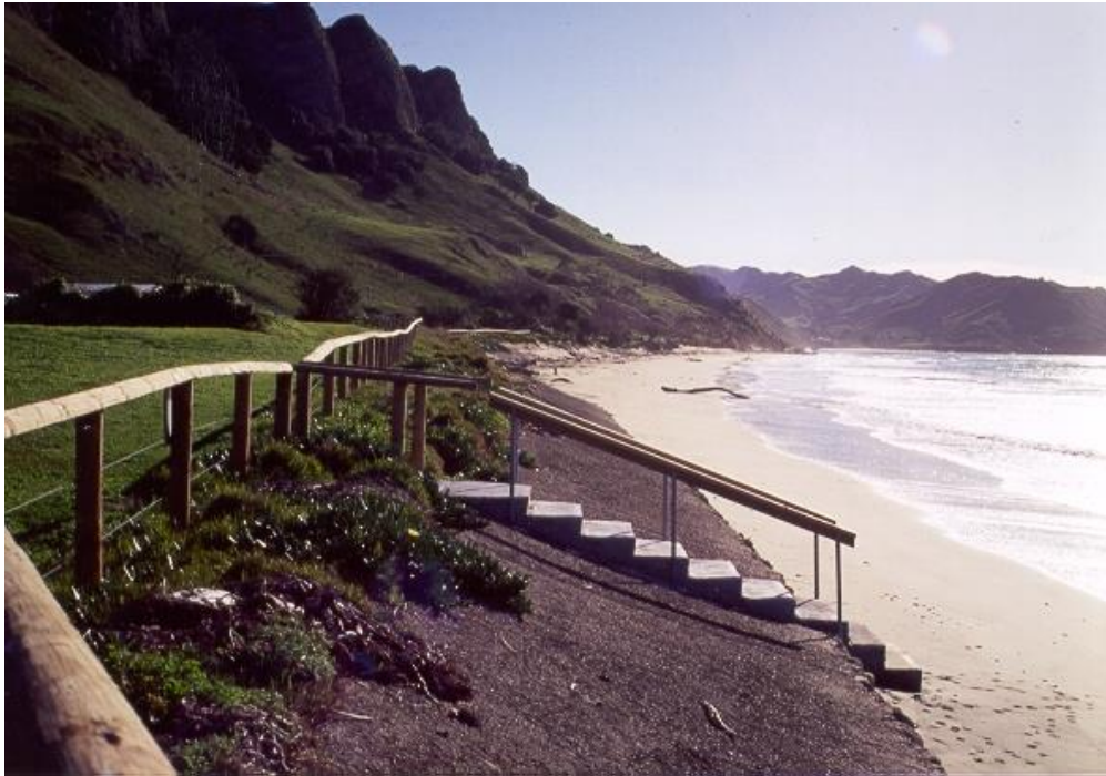
Plate 7: Armoured sections along most the Kairakau Beach has resulted in low natural character and virtually no beach at high tide. Beyond the walls toward the northern end, there may be scope to plant some native sand binders to trap sand and build up a small dune in the vicinity of scattered clumps of marram grass. Photo Sally Hobson.
