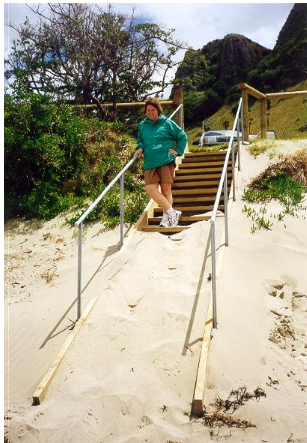
Plate 8: Recently constructed steps give access to the beach along the central portion of Kairakau Beach. Considerable movement of the fine sand since construction one month earlier covering lower steps indicates that revegetation of a zone of native sand binders could be attempted. Success will depend on a continual build of sand to create a small foredune and no storms during the critical establishment phase. Photo Sally Hobson.
