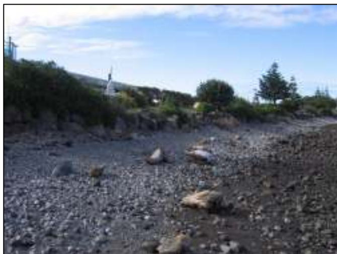
Bayly Road seawall looking south
