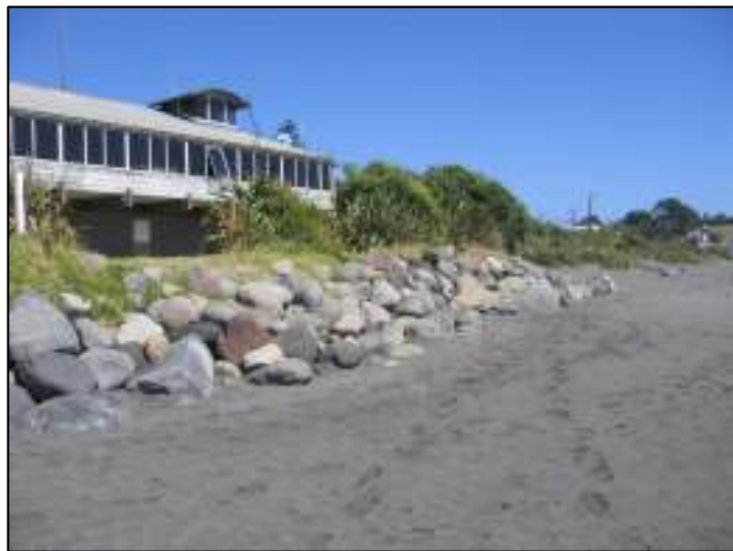
Rock rip rap protection in front of the Oakura Surf Life Saving Clubrooms.
