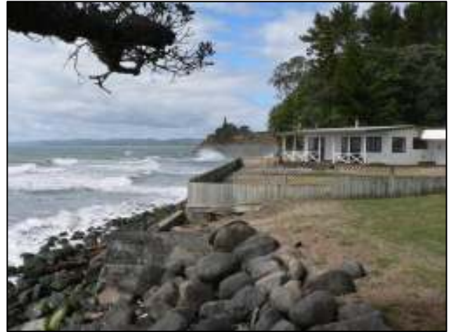
House and seawall at Onaero
