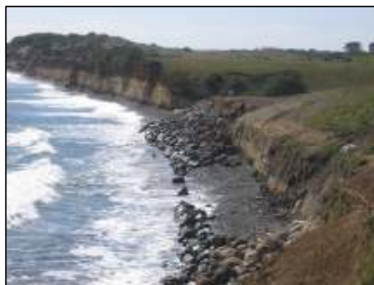
Vickers seawall at Bell Block
