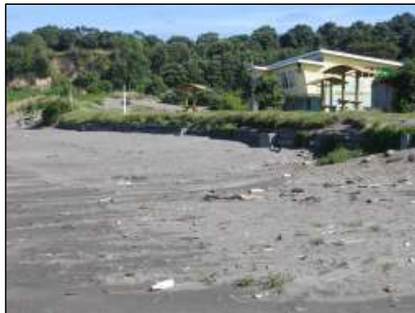
Retaining wall at Opunake Beach
