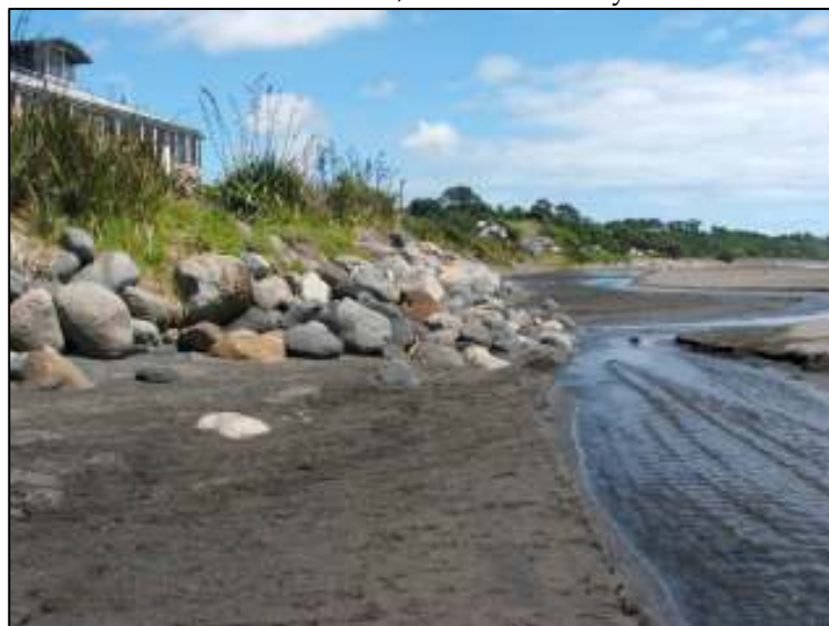
Rock protection along Oakura Beach
