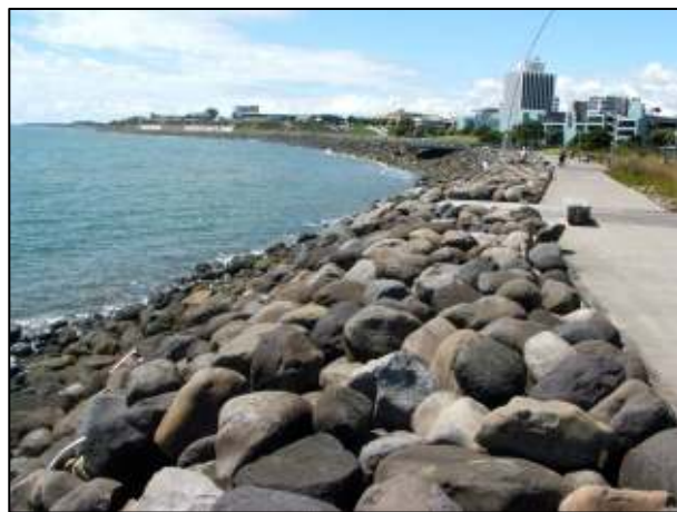
New Plymouth seawall foreshore
