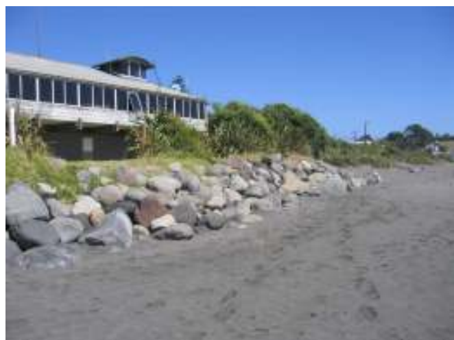
Rock rip rap protection in front of the Oakura Surf Life Saving Clubrooms.
