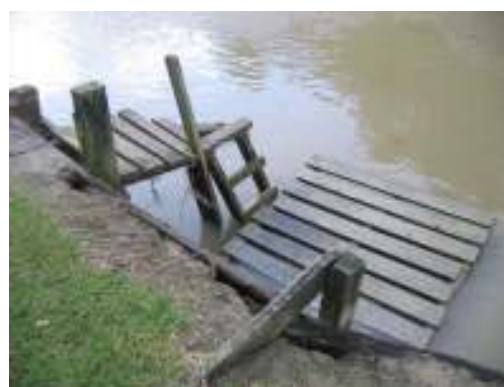
Jetties in the Onaero estuary were granted consents under B1.14, the non-complying catch all for the erection of structures in estuaries.
