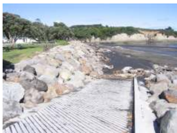
Rock wall protection at Urenui Beach.
