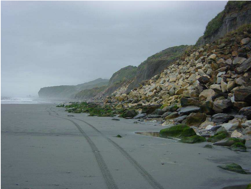
Figure 2.7 Photograph facing north displaying riprap revetments by the mudstone cliffs introduced by Transit (24/7/07)
