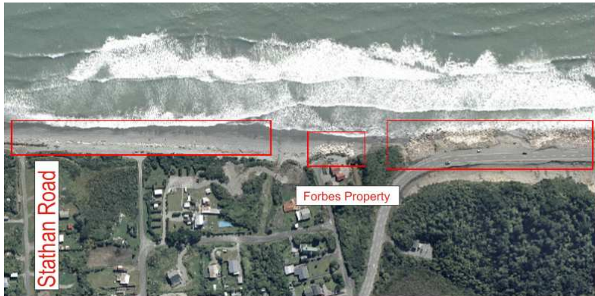
Figure 3.8 Diagram displaying the location of coastal protection (Riprap revetments) in the study area (2005)
