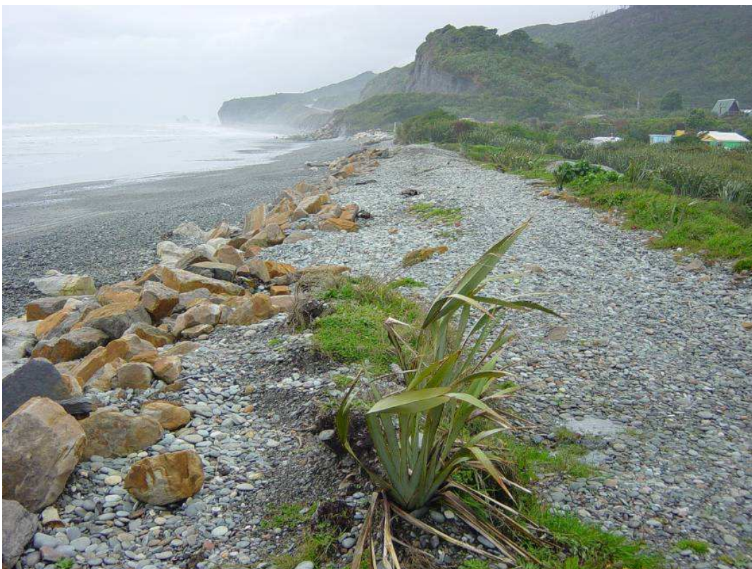
Figure 2.6 Photograph looking north displaying the riprap revetment protections along Rapahoe Beach (25/7/07)
