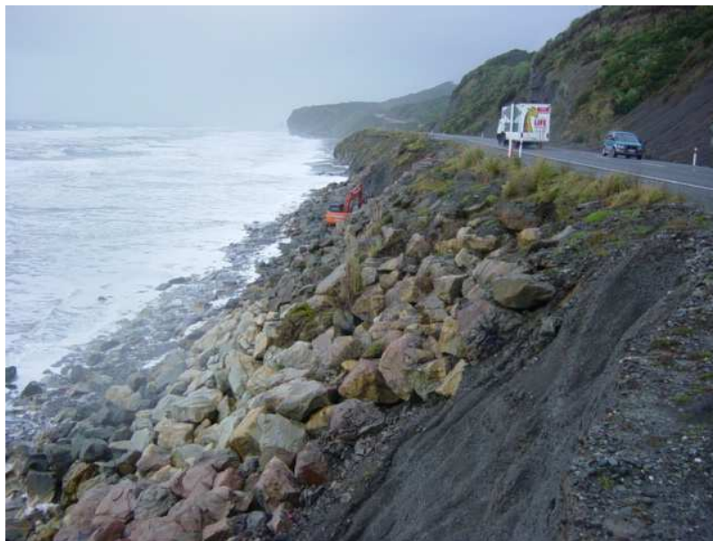
Figure 5.11 Kaiatan Cliff base undergoing revetment work at high tide
