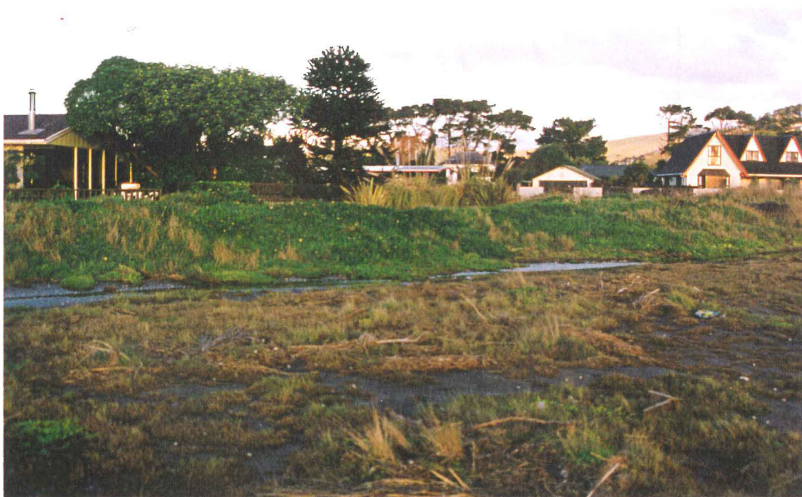
Plate 5.4 Stopbank in Front of Estuary Properties, South of Tern Street.
