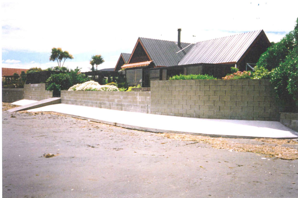
Plate 6.3 Protecting the Protective Structure - Plover Street 23 November 1994.
