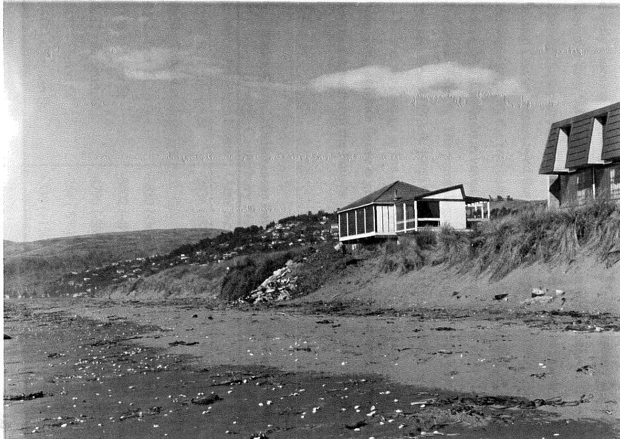
Plate 4.4 Scarp from 1977 Erosion Events - Torea Lane 1978 Note the 'protective' rubble to the left of photo and the overhang of the house (Photo: R.M.Kirk, University of Canterbury)
