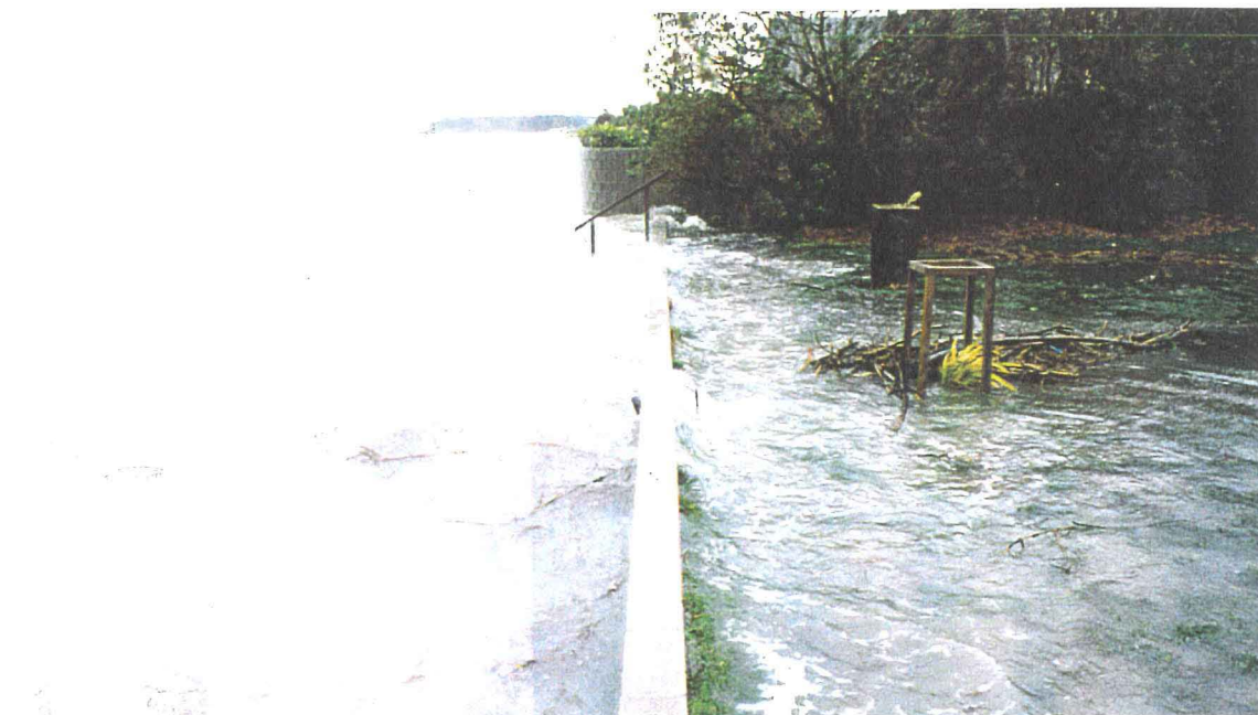
Plate 5.3 Overtopping of Seawall by Estuary at Plover Street, 29 April 1992. (Photo: Ian Ellingford, Christchurch City Council)
