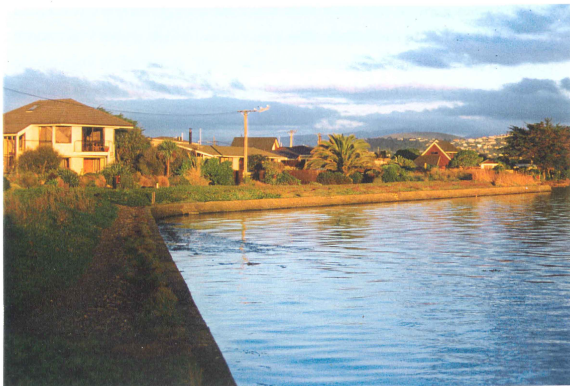
Plate 6.1 Seawall at Ebbtide Street - High Tide 27 June 1995
