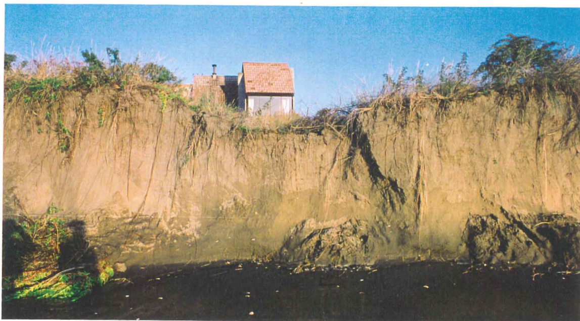
Plate 4.6 Scarp in Front of Last House on Rockinghorse Road, August 1992. (Photo: Ian Ellingford, Christchurch City Council)
