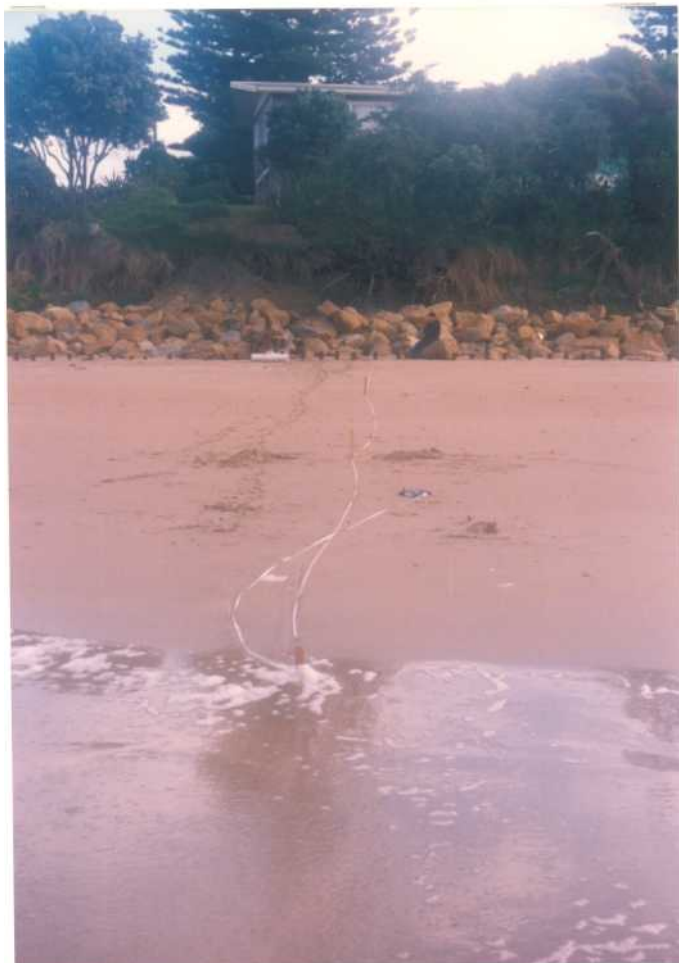
Fig. 4; View of the transect at Site B, Wainui Beach, from the low tide swash zone, The distance to the row of railway irons at the base of the protection works is 40 m.
