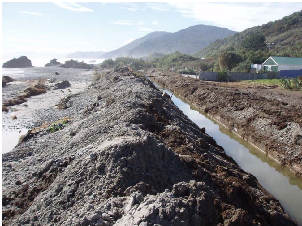
Figure 4: The re-aligned drainage channel and bund formed from the excavated material.
