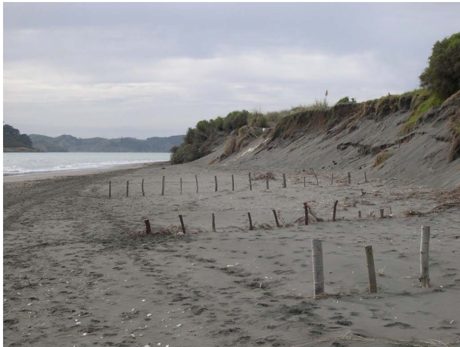
Figure 9: Use of Manuka ‘facines’ to help trap sand and raise beach levels in front of dunes at Raglan. The branches woven between the poles have now been covered with trapped sand.
