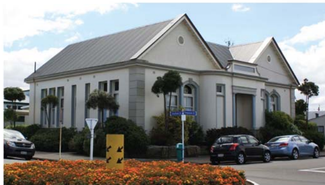
Feilding Community Centre, 21 Stafford Street (constructed 1910)
