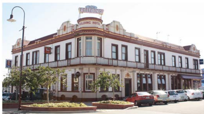
Feilding Hotel, 9 Manchester Square (constructed 1875-1910)
