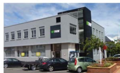
Photograph of 8 Manchester Street - (1949)
