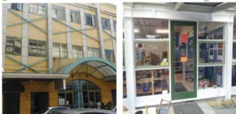
The two examples of external strengthening above contrast. The poor example (left) has cross braces (painted green) that run diagonally counter to the building's modulation. The good example (right) has a portal type bracing that fits with the door and window frame proportions and is painted the same principal white colour to de-emphasise it.
