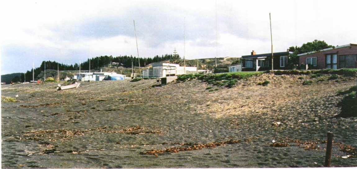
Plate 1 – View to Settlement from Beach
