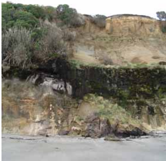
Figure 8a Cliff Slumping west of Dudley St, Orepuki, 9 September 2006
