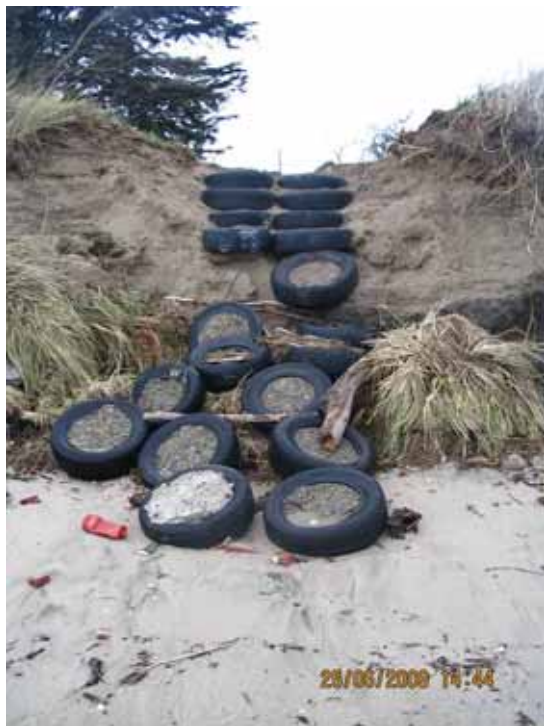
Figure 18a Recent erosion at Fortrose
