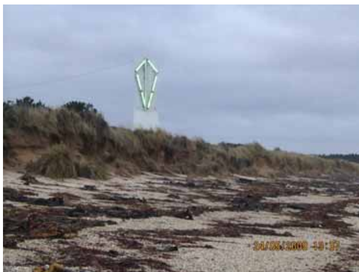
Figure 17a Bluff Harbour Leading Light, Tiwai Point
