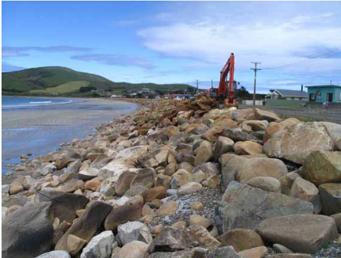
Fig 15 Rock protection under repair - 17 December 2008
