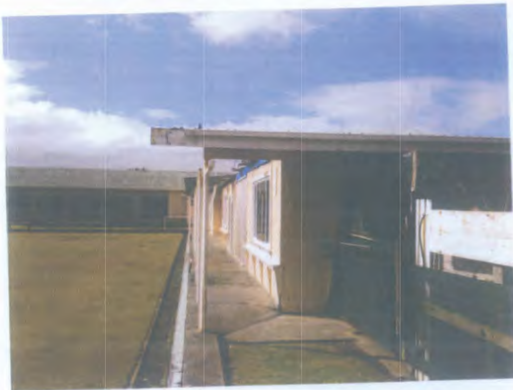
Figure 1.2: View NE showing bowling green's concrete nib (painted, centre of image), being proposed new boundary between Lots 1 & 2. Building in foreground is Women's clubhouse, with roof damage and partially boarded up. Building line is 1.58m back from proposed boundary (concrete nib).
