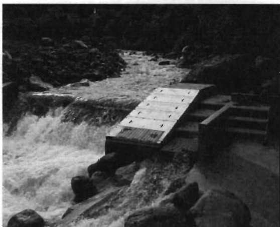
Photo caption: New fine screens at the Waimate West Water Treatment Plant
