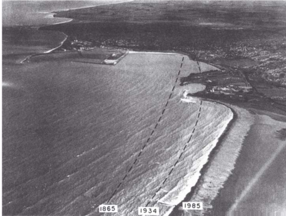
Figure 6-8 A 1985 oblique aerial photograph of the eroding Washdyke Beach, with the positions of the pre-breakwater 1865 shoreline and that in 1934 surveyed about 40 years following the breakwater construction. [from Kirk (1992b)]
