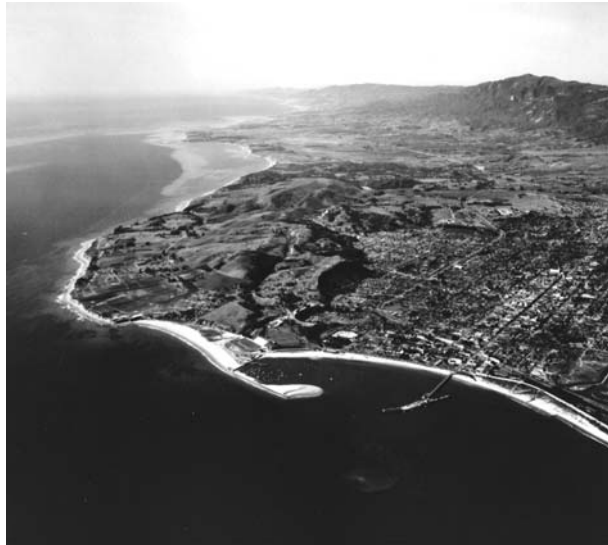
Figure 6-5 The Santa Barbara breakwater, California, with sand accretion on its updrift side and within the harbour entrance as a spit of sand. [Photo courtesy of Prof. Robert Wiegel]
