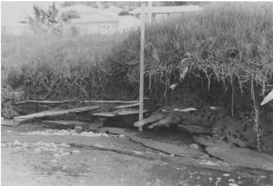
Fig. 3—Photograph showing the eroding reclamation of kauri sawn planks in a matrix of sawdust and wood chips exposed above high water mark near Bay Vue Road, Tairua. Plank orientation suggests that the slabs have been systematically laid rather than dumped (rule is one metre). Photo taken on 14 May 1984.
