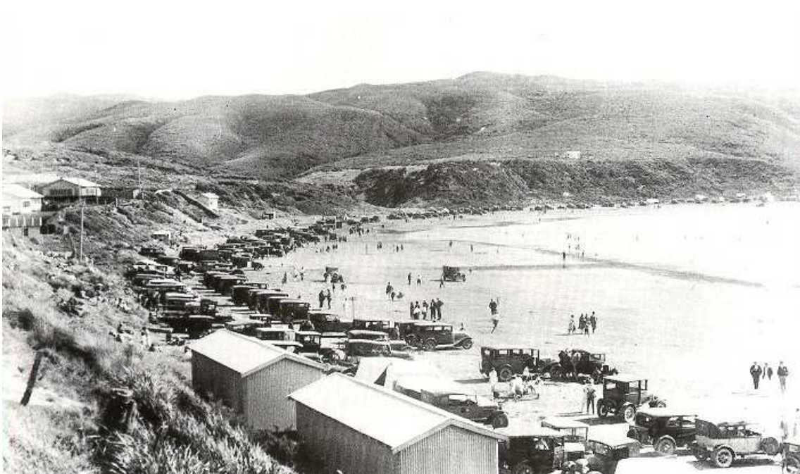
Figure 8. Titahi Bay circa 1920. Vegetation had been cleared from the back and foredunes. What appears to be Marram can be seen in the foreground behind the boat sheds. Buildings had been constructed on the top of the foredunes. Even at this stage, vehicles played a prominent role in recreation on the beach.
