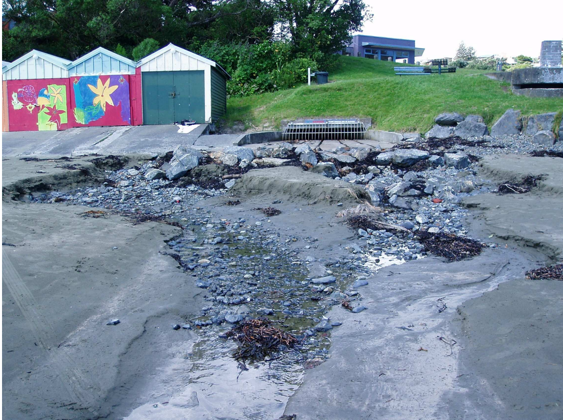
Figure 9. Stormwater outfalls, like this one at the northern end of Titahi Bay, have an adverse effect on sandy beaches, causing scouring and making the beach extremely vulnerable to erosion from wave run-up.
