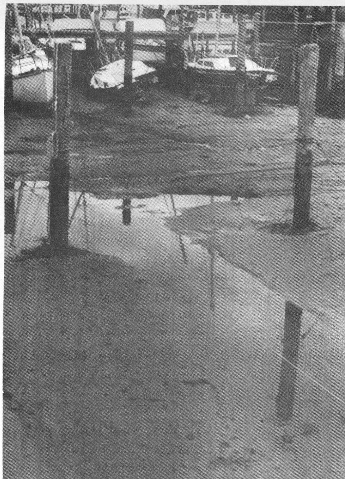
Plate 4.1 : Build-up of muddy sediments in the berthage areas on the western side of the Milford Marina. Note the keel drag marks and holes scoured by propeller wash. Photo taken on 2 May 1980.
