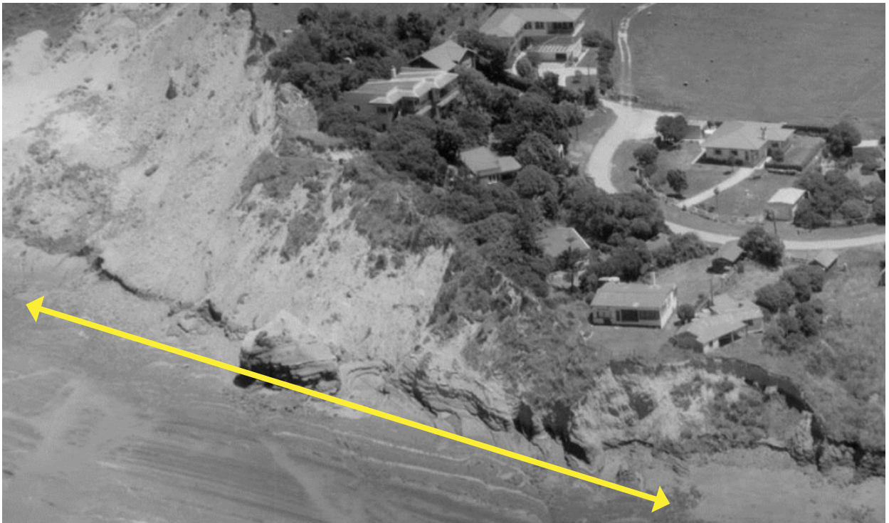
Figure 3 View of Area 2 (and northern part of Area 1) in December 1955 showing the natural character and erosion/landslide mechanisms in this area prior to placement of erosion protection works. Note: Double-headed arrow shows approximate longshore extent of Area 2 (Source – Alexander Turnbull Library in Tonkin and Taylor and Eco Nomos, 2013)
