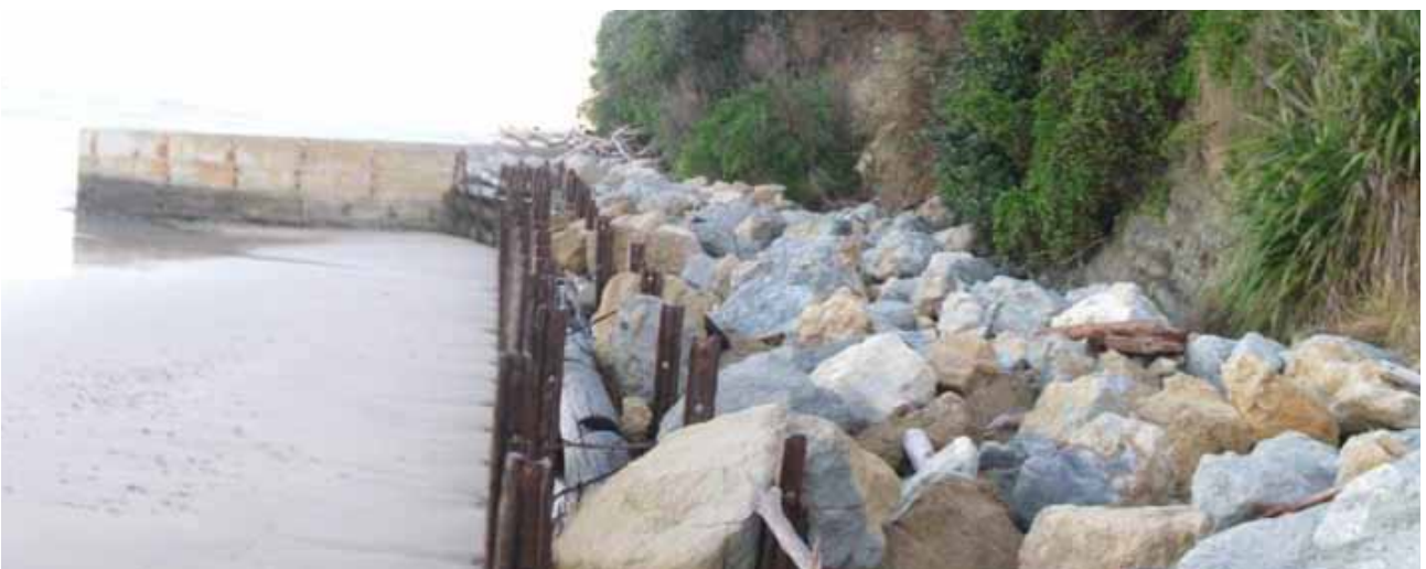
Figure 4: View of recent rock revetment in constructed south of the groyne in Area 2 (top) and the historic works south of the groyne (bottom). (Source: Photo taken July 2013, Tonkin and Taylor and Eco Nomos, 2013)
