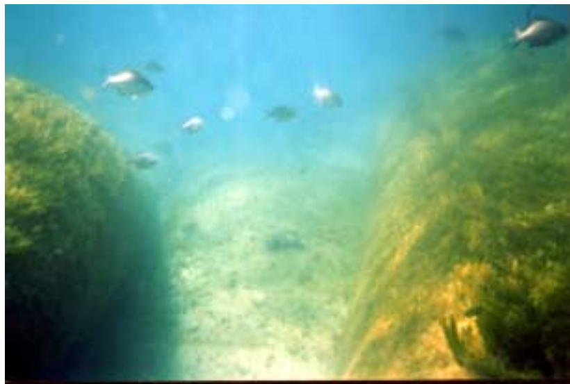
Figure 7.5. After 18 months on the seabed, the geotextile containers that comprise the Narrowneck Reef on the Gold Coast are a flourishing habitat in a relative ‘desert’ of mobile sand.
