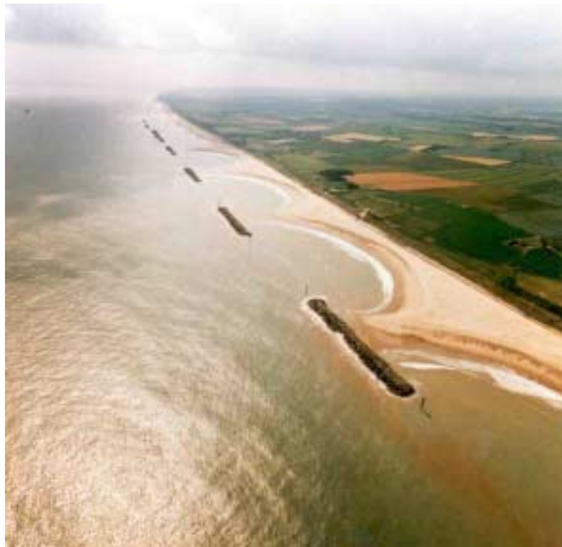
Figure 7.3. An example of a detached breakwater project in East Anglia, Great Britain. Note the formation of tombolos in the lee of the breakwaters. The sand was placed as nourishment, not trapped from the natural system.
