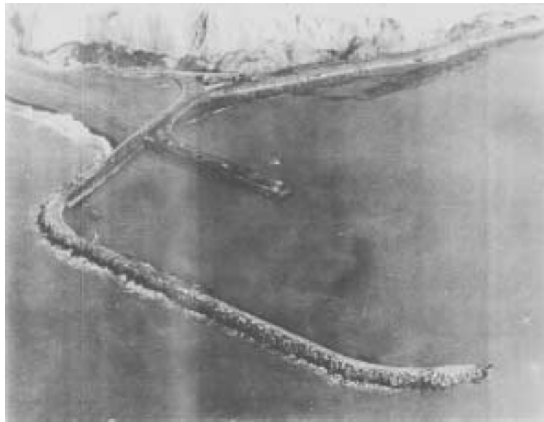
Figure 3.3. Early Port construction (circa 1933) – note the large build-up of shingle/sand on the southern side of the works (upper left-hand side).
