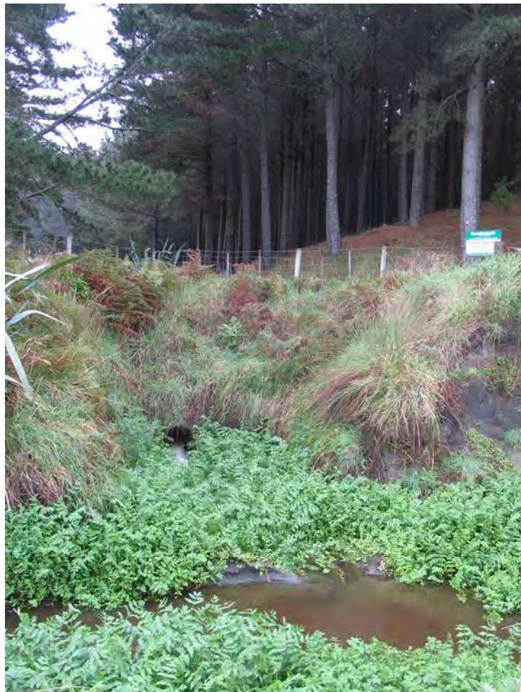
Figure 4. A drain outflow diverting surface water, from land irrigated with treated effluent, into the Waiwiri Stream.
