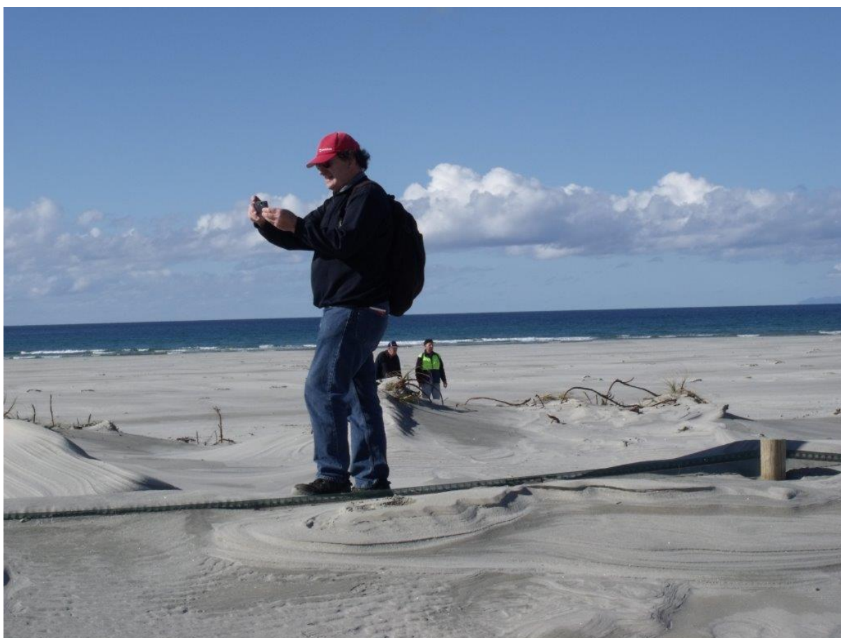
Photo 6. Top of sand fence exposed by heavy storms. Note lack of sandbinders following heavy storm erosion, but buildup of sand around surviving vegetation and other obstructions on the beach.
