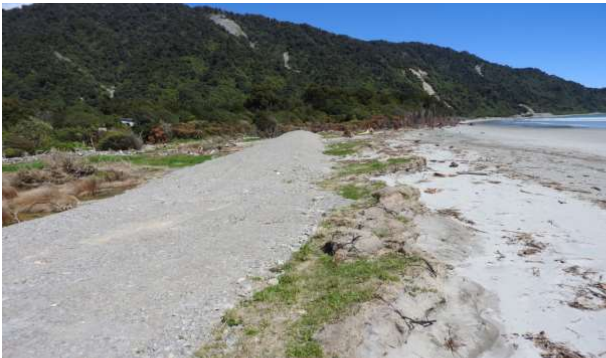
FIGURE 1 PHOTOGRAPH OF THE EMERGENCY SACRIFICIAL BUND THAT HAS BEEN ESTABLISHED
