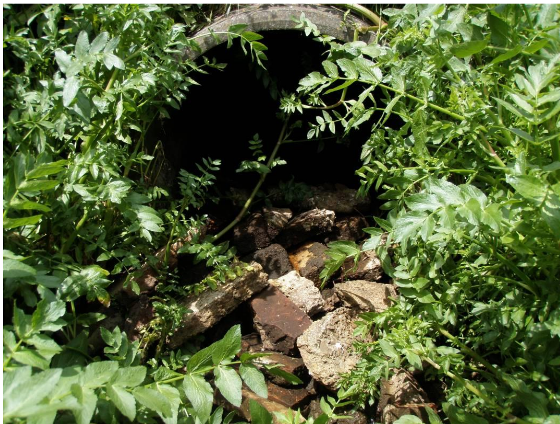
Plate 7: Culvert mouth, Wairarawa Stream.
