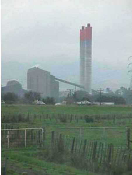
Huntly Power Station
