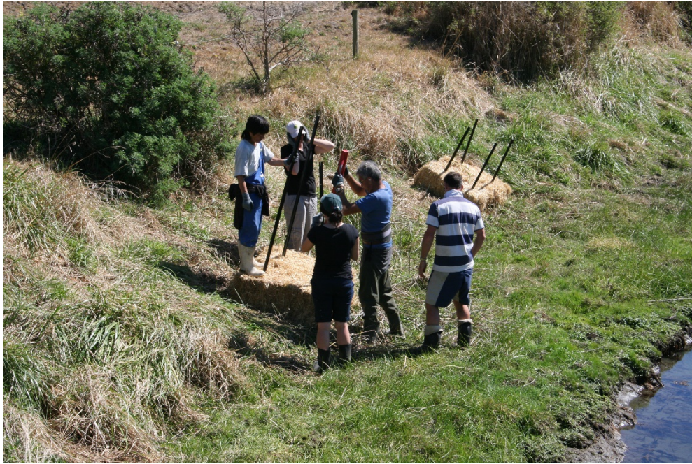
Figure 5. Straw bale installation within the Ōhau Loop with local kaitiaki.
