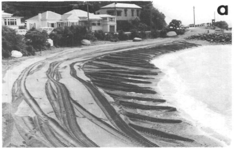
Fig. 6 Sequence showing the establishment of the beach face and berm just 16 days after dumping and mechanical grooming of nourishment sediment. Photograph a taken 18.10.82, b taken 21.10.82 after weak southerly wave attack ( H_{1/3} = 0.1 m, T_{1/3} = 1.2 s), and c taken 3.11.82 after gale-force northerly winds when waves were H_{1/3} = 0.7 m, T_{1/3} = 3.25 s.
