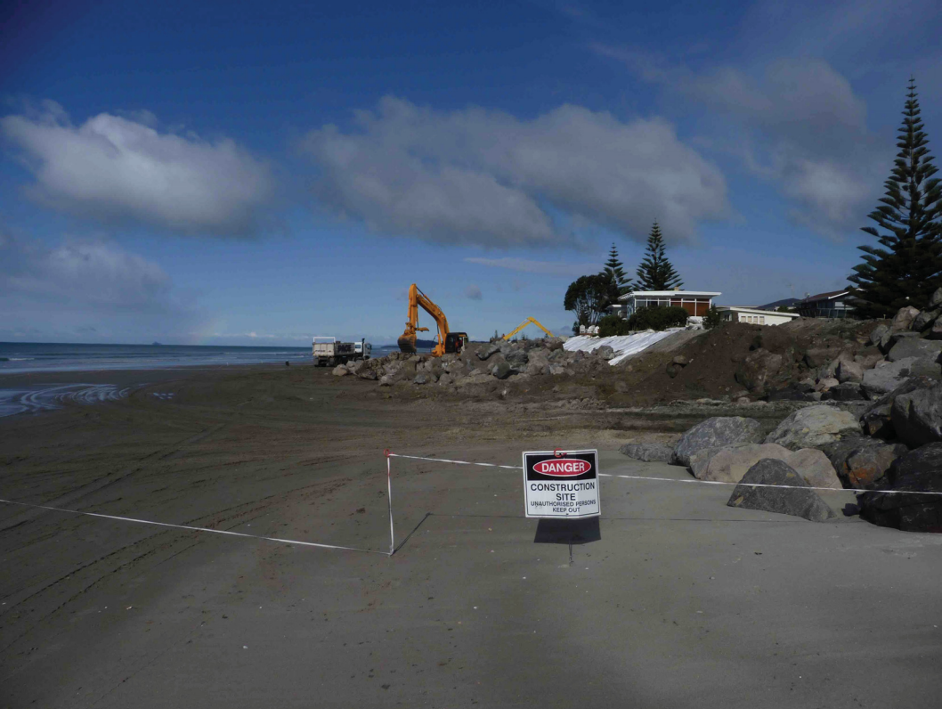
Fig. 6: Construction of the seawall. Picture by author, September 2011.
