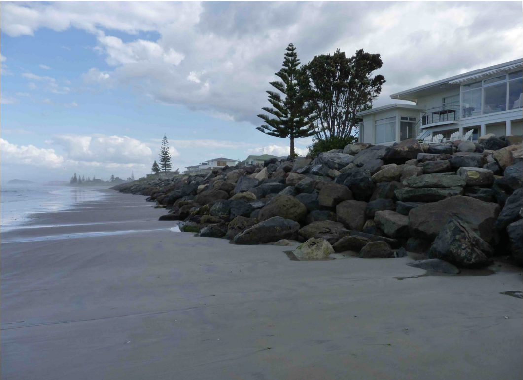
Fig. 7: The new seawall at low tide. Picture by author, March 2015.
