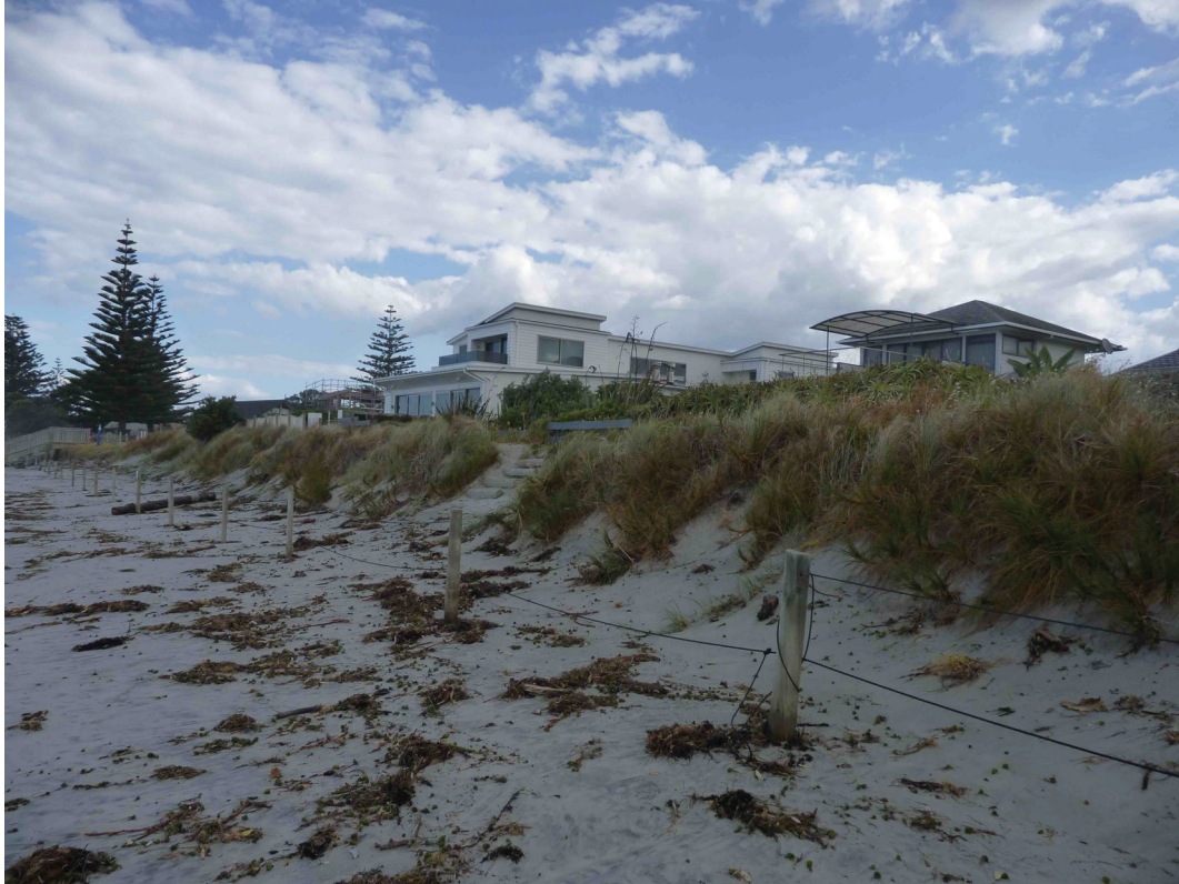
Fig. 11 and 12: Waihi Beach dune enhancement, four years later. The sandbags have been added in some parts as a “temporary access structure”. Pictures by author, March 2015
