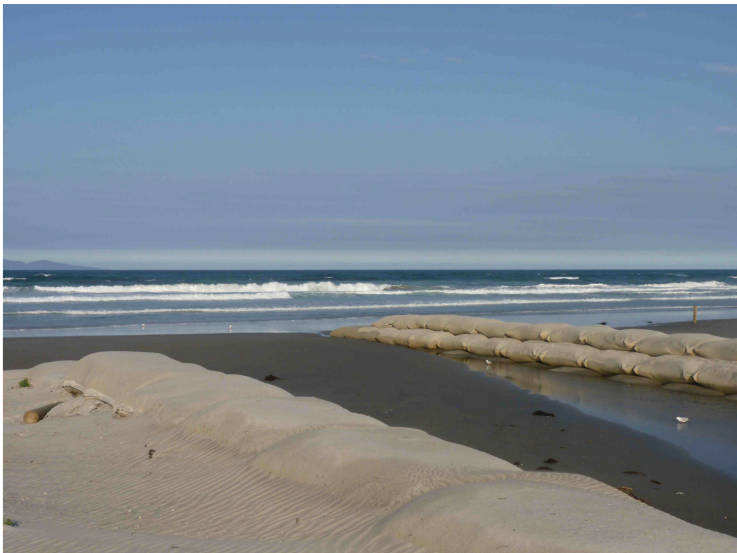
Fig. 5: Waihi Beach, Three Mile Creek training with geotextile bags. Picture by author, December 2010.
