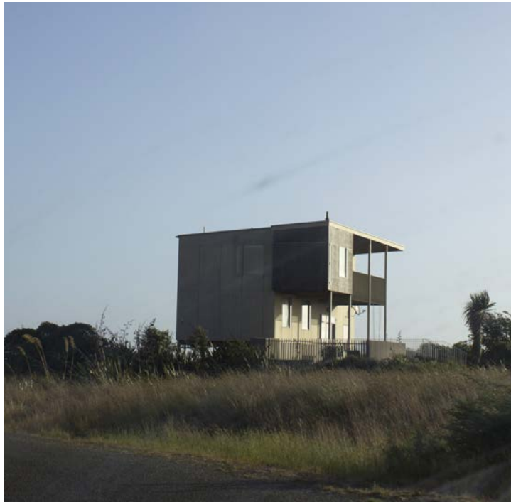
Fig. 39 Many of the beach houses and lifestyle blocks are situated on large, almost empty lots.
