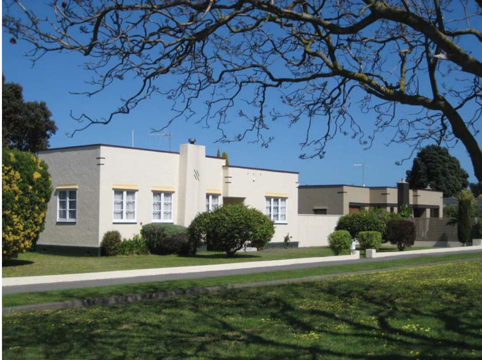
Figure 6.14: Art Deco houses in Georges Drive, in the 28-Acre Block, Mārewa.
