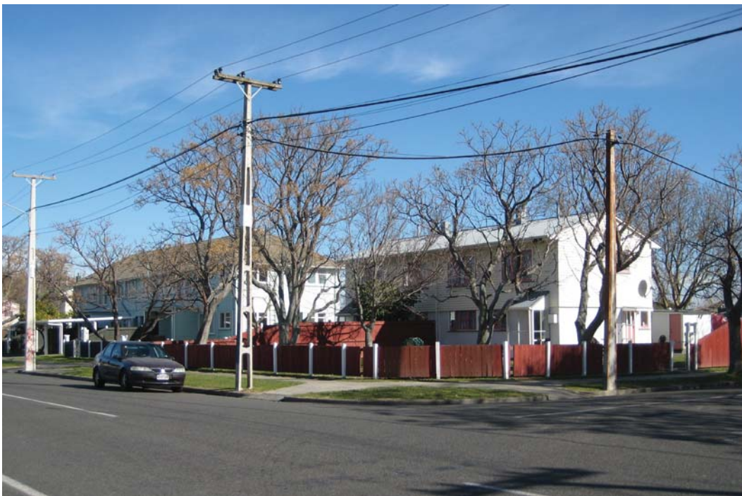
Figure 6.12: State Housing, multi-unit accommodation in Bledisloe Road, Maraenui.
