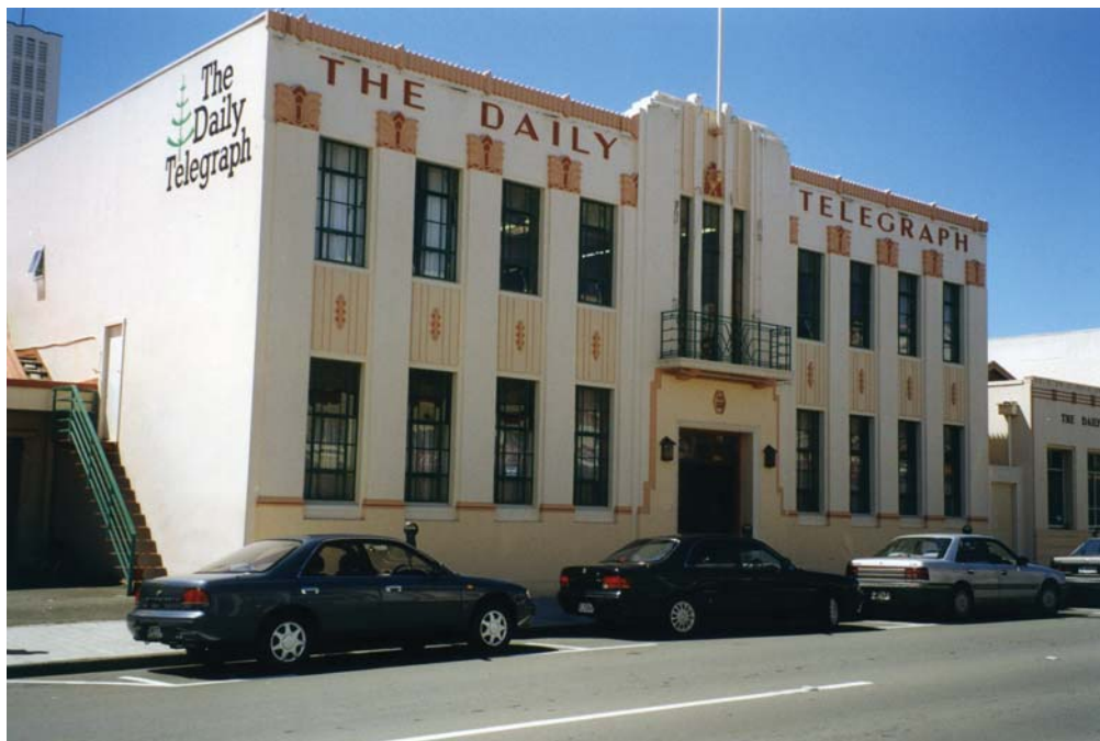
Figure 5.10: Daily Telegraph Building, Tennyson Street.
