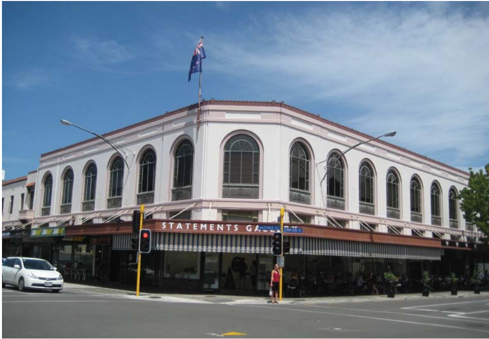
Figure 5.9: Market Reserve Building, Tennyson and Hastings Streets, the first significant post-earthquake building.
