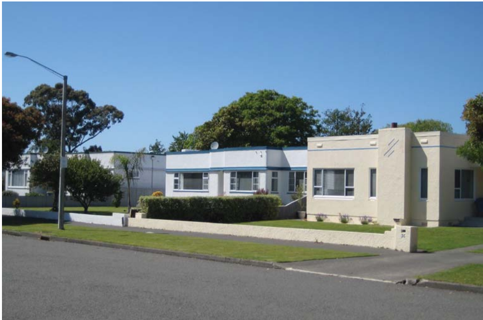
Figure 6.15: Art Deco houses in Logan Avenue, in the 28-Acre Block, Mārewa.
