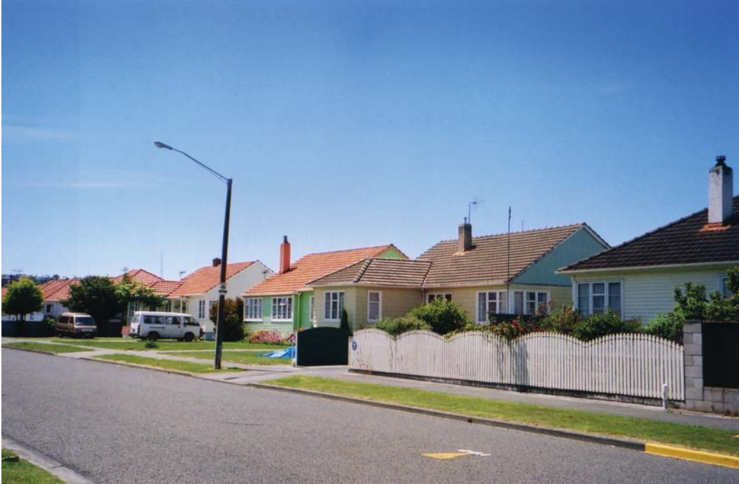
Figure 6.11: State Housing, single unit accommodation in Russell Road, Marewa.
