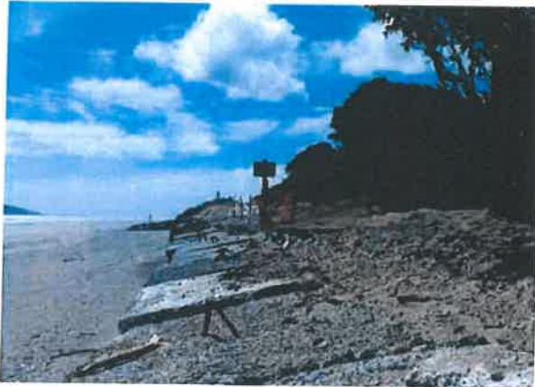
Figure 2 Crest of existing block wall
