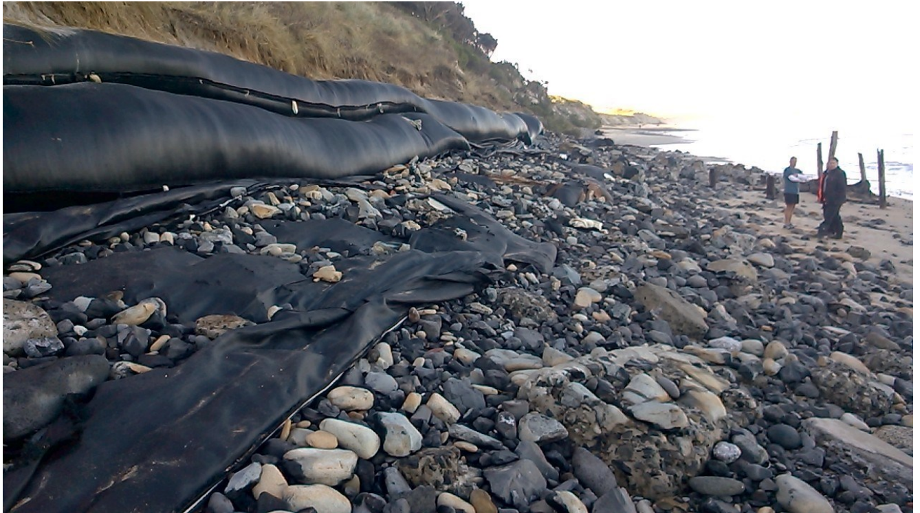
Photograph 1 Geotube backstop wall
