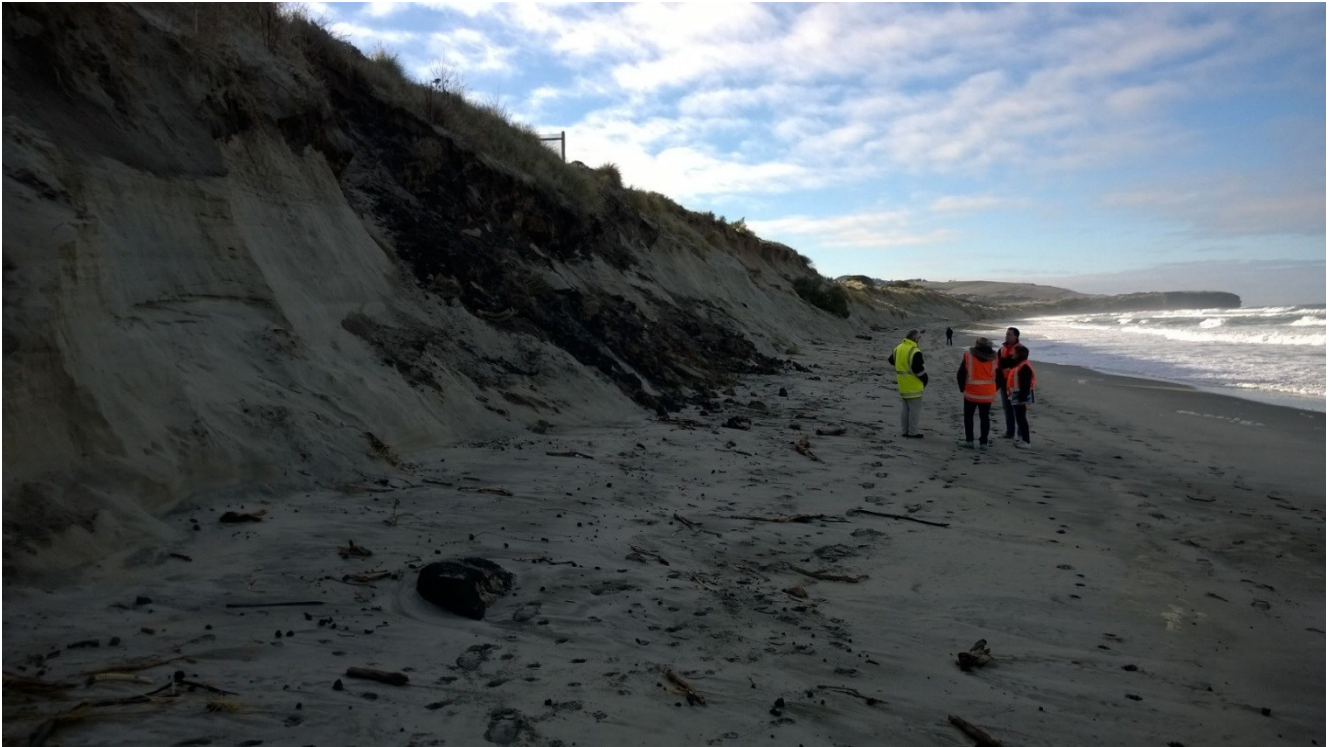
Photograph 3 Construction debris on eroded dune face
