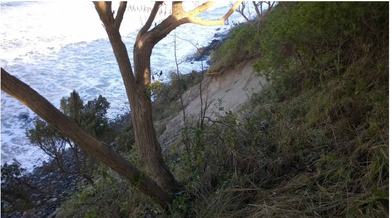
Photograph 4 Erosion of the dune face to the east of the geotube wall
