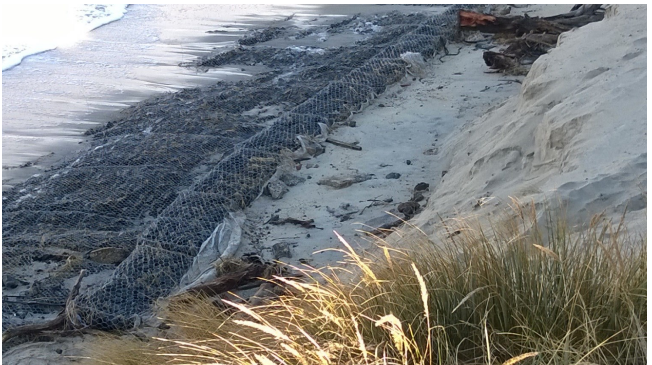
Photograph 2 Reno mattress toe
